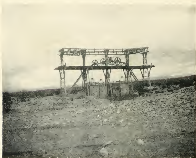
FAMATINA MINE—TENSION STATION OF AERIAL ROPE-WAY.
